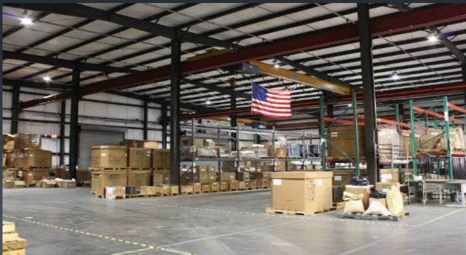
APL in a Factory (Los Angeles, California)
